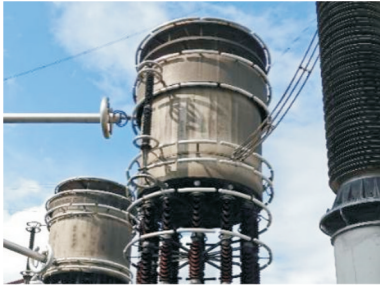
图1 PKK-800-5000-50G 型电抗器实物图 Fig. 1 Photograph of a smoothing reactor PKK-800-5000-50G
